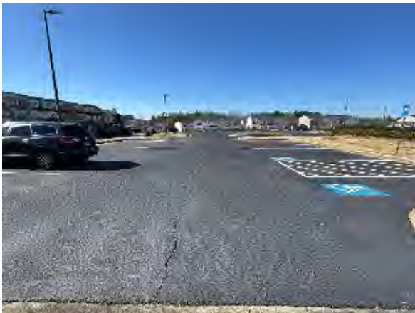
Parking Lot View
