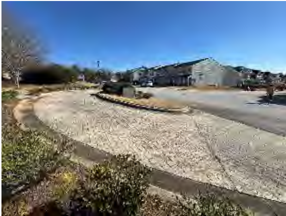
Stamped Concrete Cul-de-sac Turnaround
