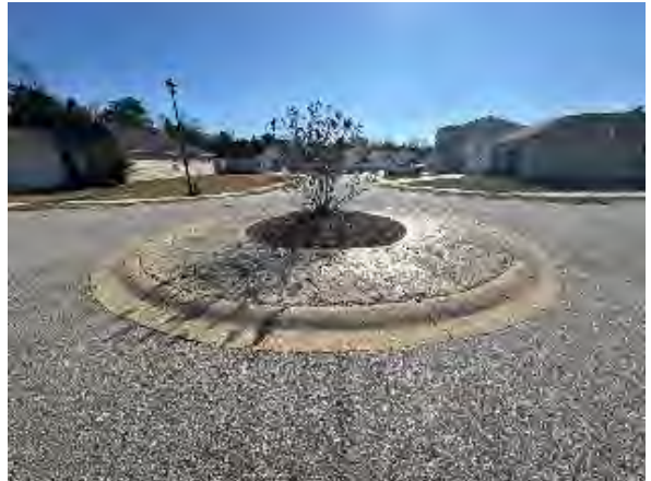
Stamped Concrete Traffic Island
